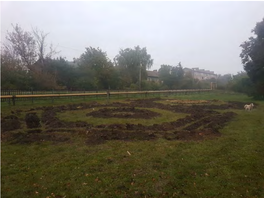
Fig. 8. Earth works on establishing an Intensive Food Forest (MIFF) Module
