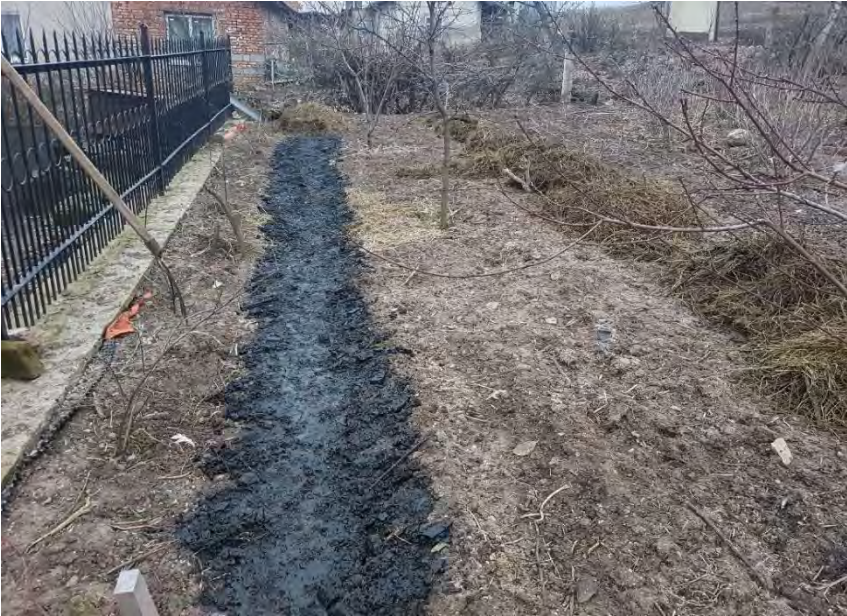
Fig. 7. Placing the biochar in the WRB
